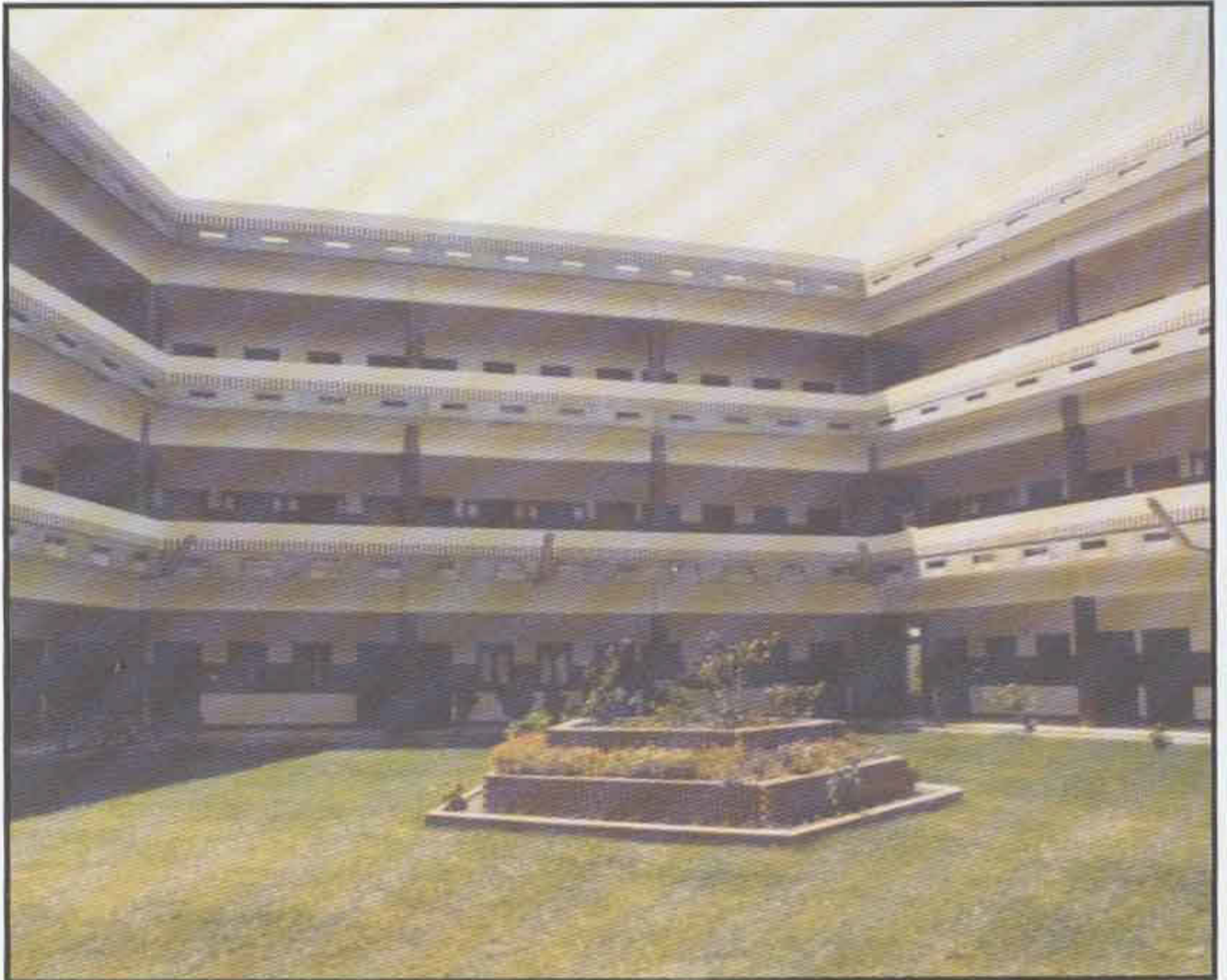
Interior View of the Impressive three Storied of New Classrooms
